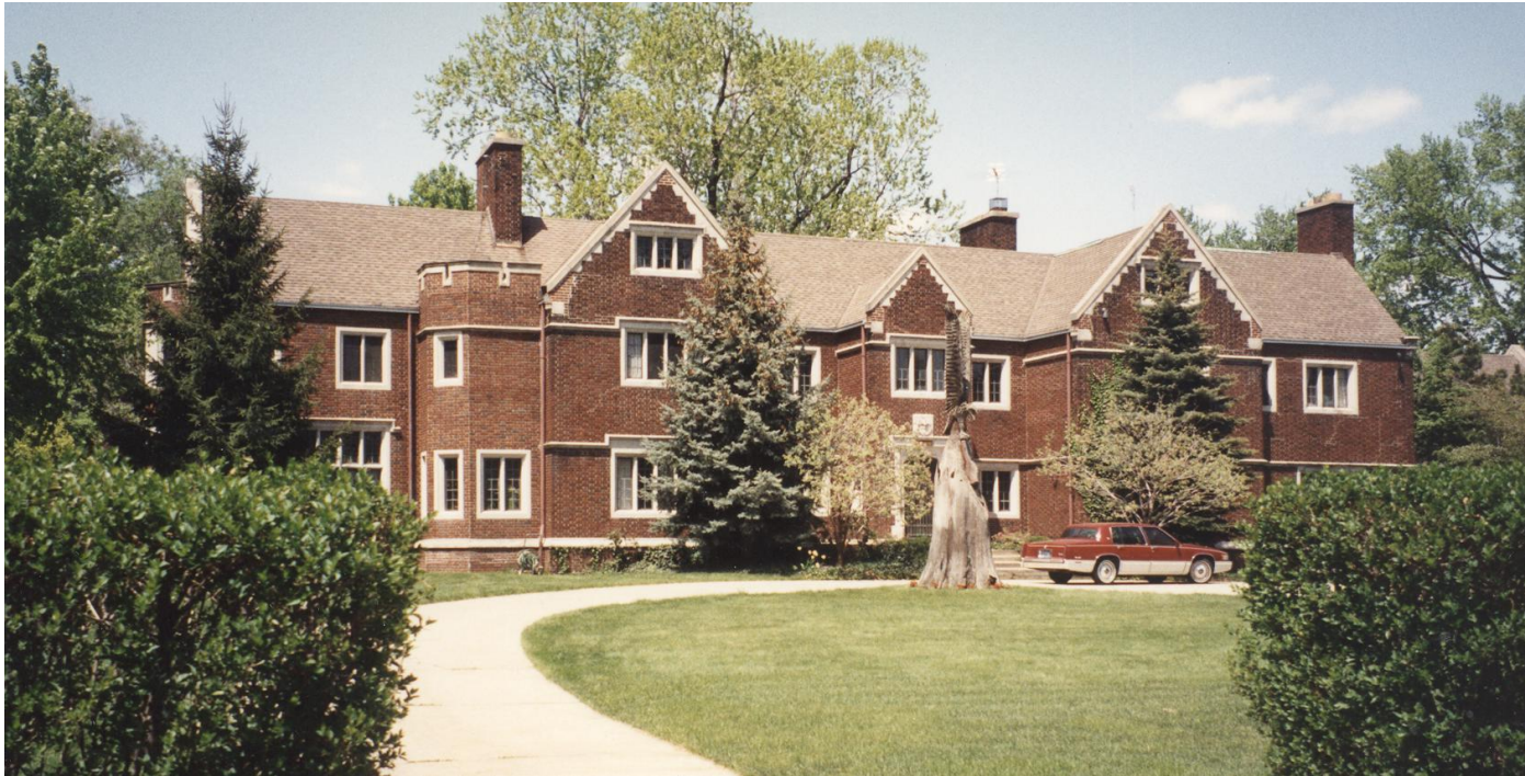
Lawn Leighton 16761 E. Jefferson Avenue Grosse Pointe Park, MI 48230 Built: 1915 Architect: Louis Kamper Style: Tudor Revival
