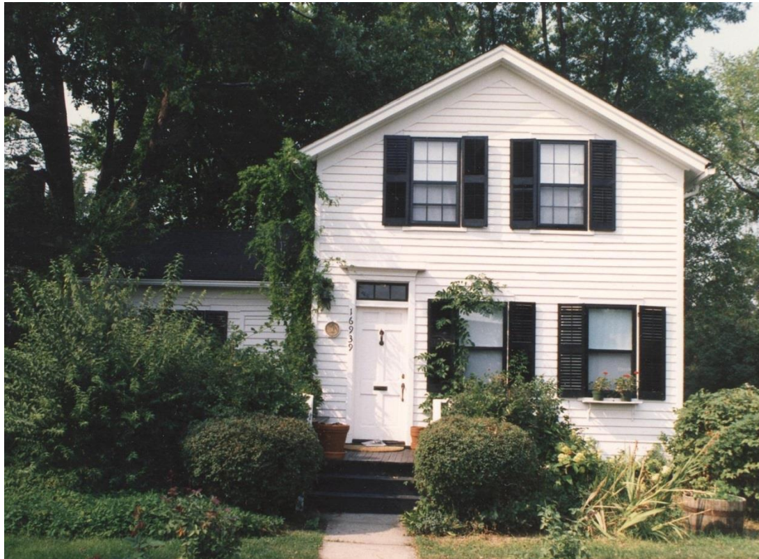
Isidore Cadieux Farmhouse Moved to 533 St. Clair in 2014 Grosse Pointe, MI 48230 Built: 1866? Style: Farmhouse Clapboard
