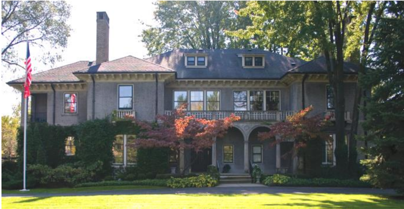
1 Rathbone Place Grosse Pointe City, MI 48230 Built: 1918 Architect: Louis Kamper Style: Elements of the Romanesque Revival and French Classical Revival styles
