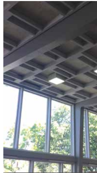
Ceiling detail, Central Branch Library (1955)
